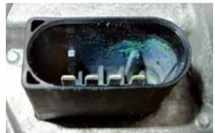
Built-in plug with traces of corrosion
